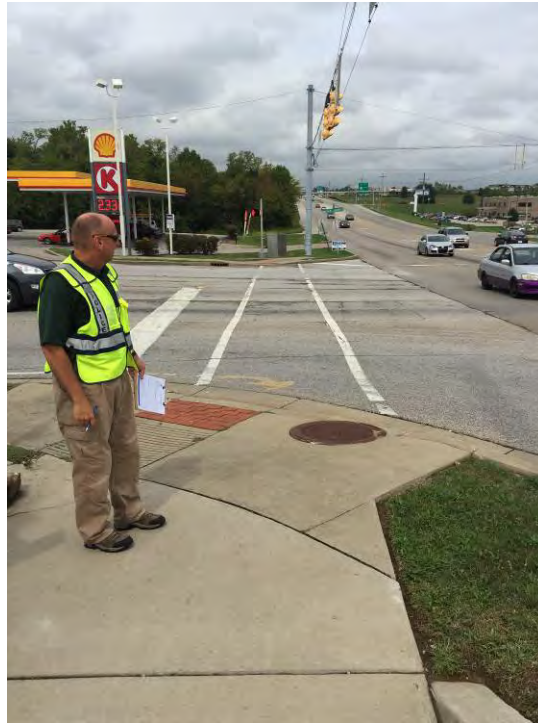
Photo 24: Consideration of the length of the Pedestrian phase is needed at long crosswalk locations.
