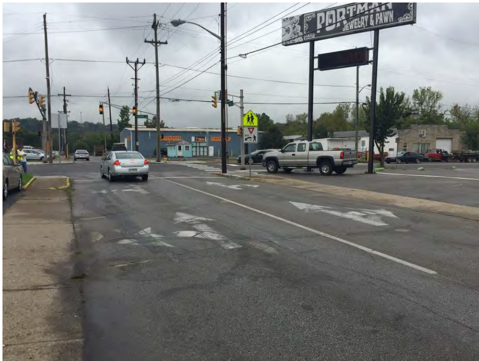
Photo 19: This is an example of where directional pavement markings without overhead signs, can lead to driver confusion.
