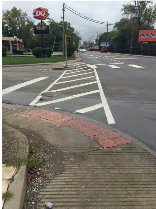
Photo 1: State at Cherry PED Xing illustrates the value of upgrading PED Islands. Here pavement markings have been enhanced to provide better definition of the pathway.
