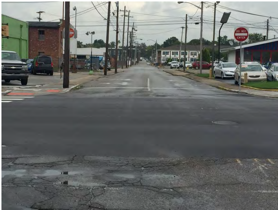
Photo 17: Pavement surface is smooth through the mainline, but the transition to worn pavement on a minor volume street can be seen here.
