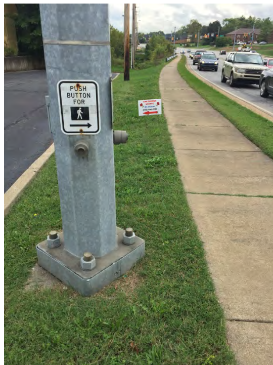
Photo 29: Pedestrian push buttons need to have sidewalk extensions and/or relocation to align with the Pedestrian Indicators to ease crossing.
