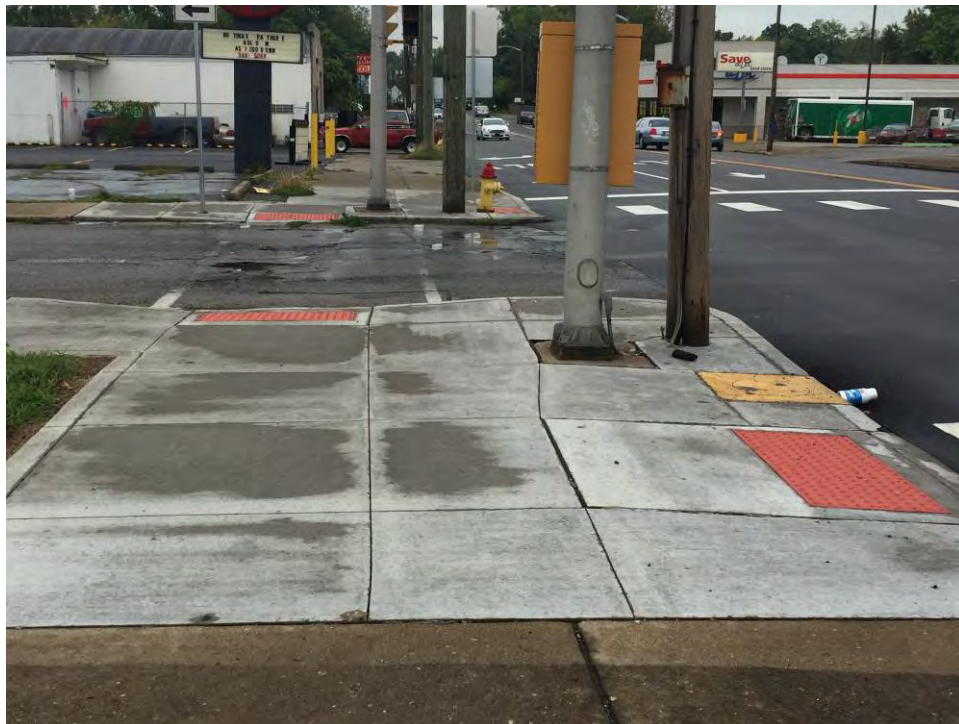
Photo 9: Upgrades to Pedestrian Crossing ramp slopes and turning spaces need to be partnered with providing close access to Pedestrian buttons.
