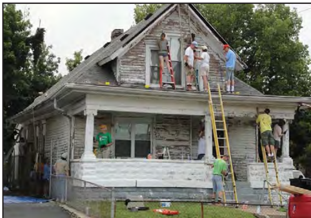
Home rehabilitation efforts Source: New Direction Housing Corporation
